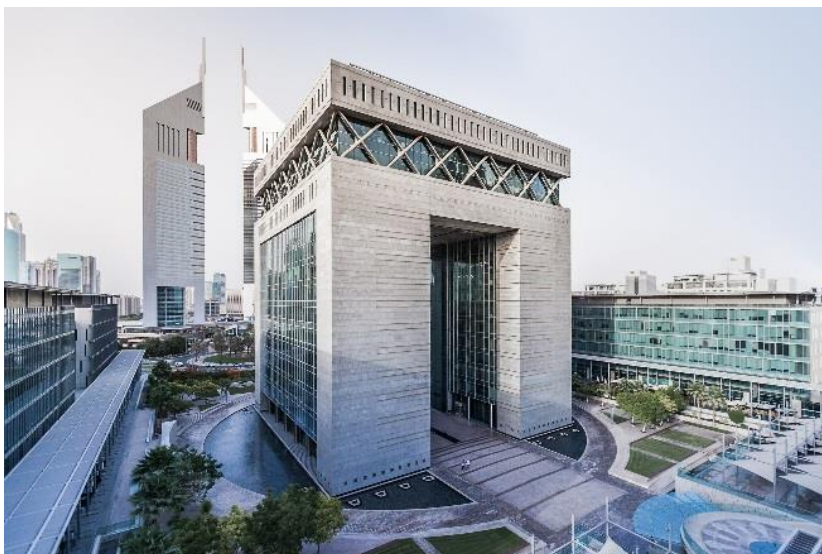
The Access Bank UK DIFC Branch situated in the iconic Gate Building of Dubai International Financial Centre.
