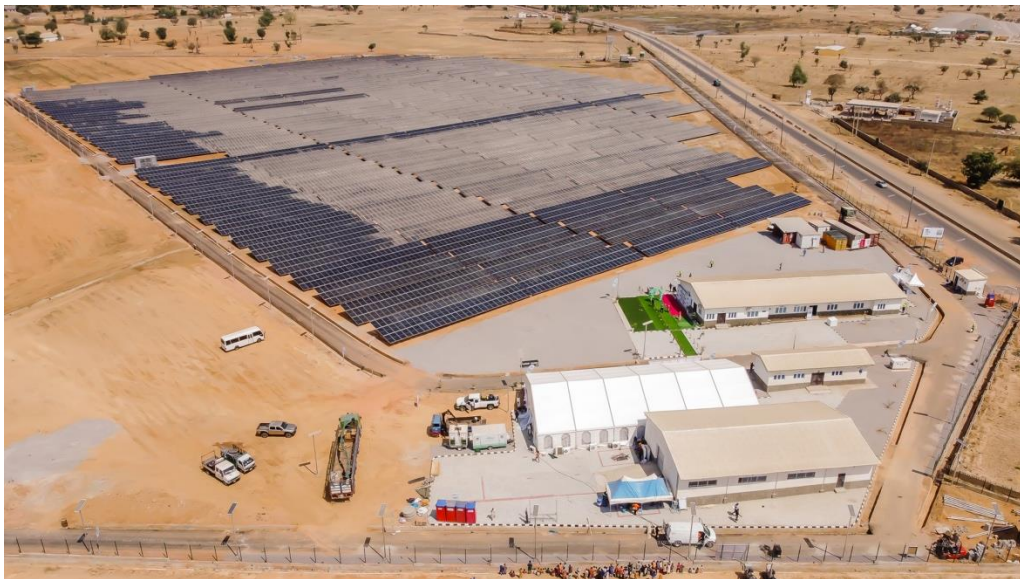
Figure 1 Aerial footage of the PV array
